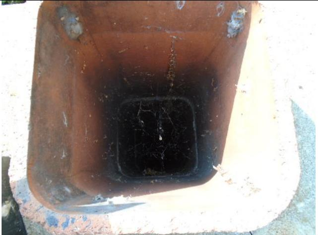
Interior view of unlined masonry chimney. We recommend liners for all chimney applications be installed by a licensed professional to ensure the appropriate flue liner material is used for each application.
