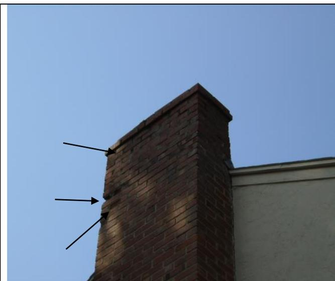
Spalling occurs when brick deteriorate and layers 'flake off' causing damage.
