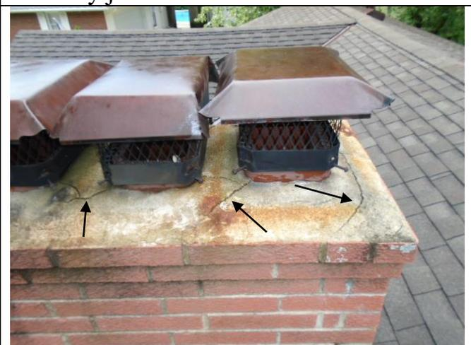
Cracks in chimney caps should be sealed brush on elastomeric sealant for long term protection. This covers the entire chimney cap and provides a waterproof seal.
