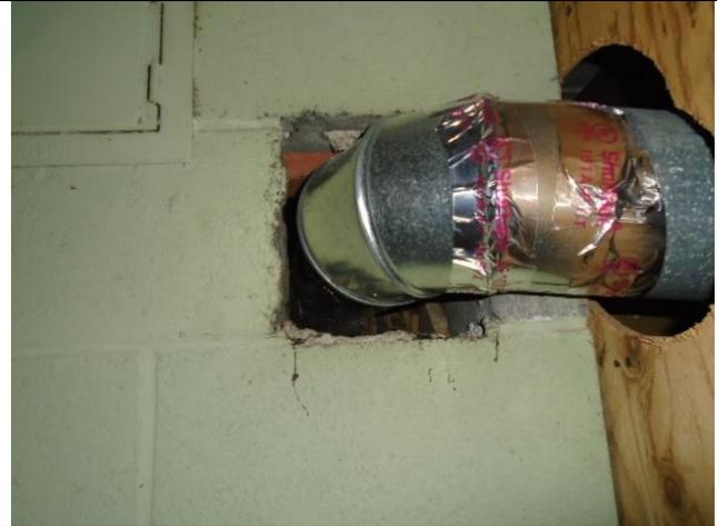
This photo shows a gas appliance flue discharging into an open masonry chimney; this has a high potential for flue gasses to leak back into the home due to pressure differential and down drafting.
