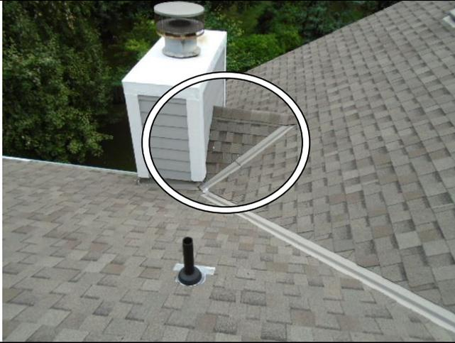
A chimney cricket is a 'peak' at the center of the chimney base that diverts water and minimizes the potential for snow accumulation. A cricket, as shown here, is recommended for any span over 30 inches.
