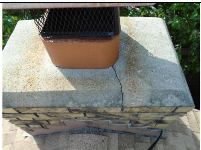
Some cracks are large enough that you can apply a polyurethane caulking to fill cracks prior to applying the brush on sealant.
