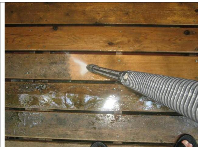
Hold the spray nozzle about 12” from the wood and have the nozzle adjusted to fan out about 6” wide. Hold the wand at an angle, and keep the wand moving.
