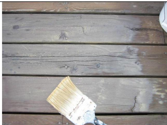
Apply a thick coat of sealant with a stain pad applicator or 4” white china brush.
