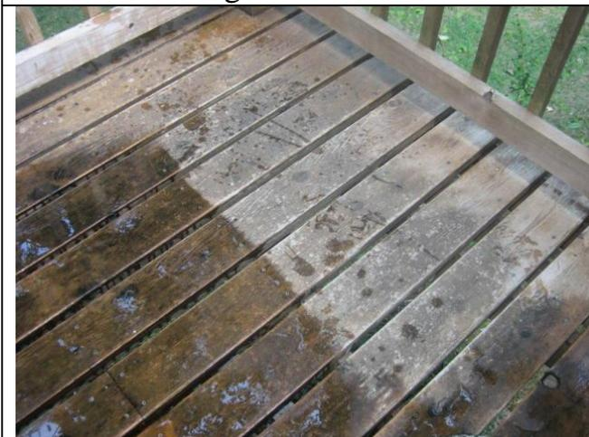
If the deck is in good condition but dirty you can power wash the deck prior to applying the sealant. This will ensure the sealant penetrates the wood properly.
