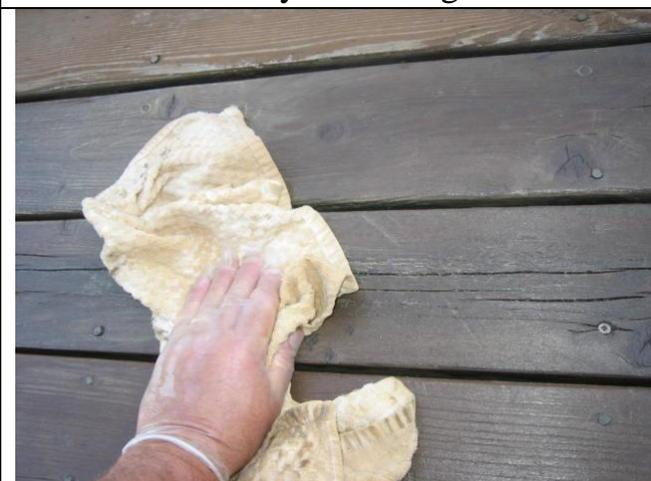
After application with a brush, rub the sealant in with rag to get better penetration and minimize wet spots.
