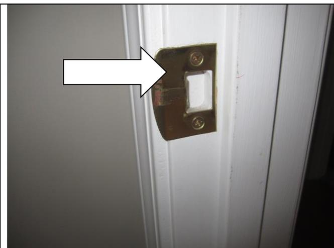
If the latch is missing high on the strike-plate insert the 3 inch screw in the lower hinge center hole.
