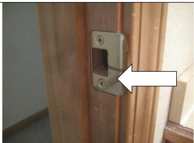
If the latch is missing low on the strike-plate insert the 3 inch screw in the lower hinge center hole.
