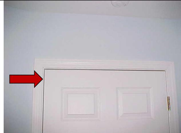
If the door sticks at the “top-top” insert the 3 in screw in the lower hinge center hole.
