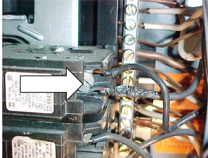
Double lugging is a commonly identified condition observed during inspection of a homes main electric panel. This refers to a connection where two circuit wires terminate under a single lug within the main electrical panel. Problems occur when one of the wires under the lug is not secure or the maximum load is exceeded on a breaker.
