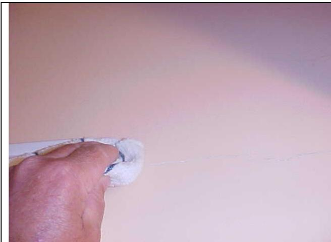
Use a damp rag to wipe off excess spackling; try not to remove any from inside the crack, a smooth finish is best.
