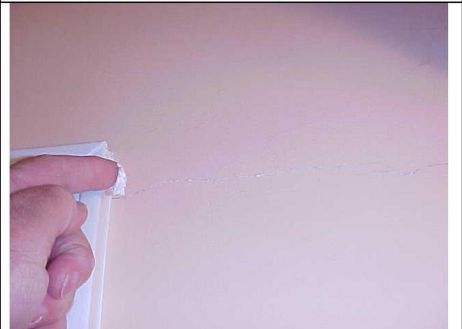
This crack is large enough to be noticed but also easily repaired with spackling.
