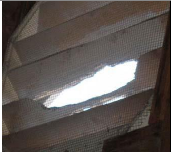
From inside the attic you can see the screen mesh has been torn.
