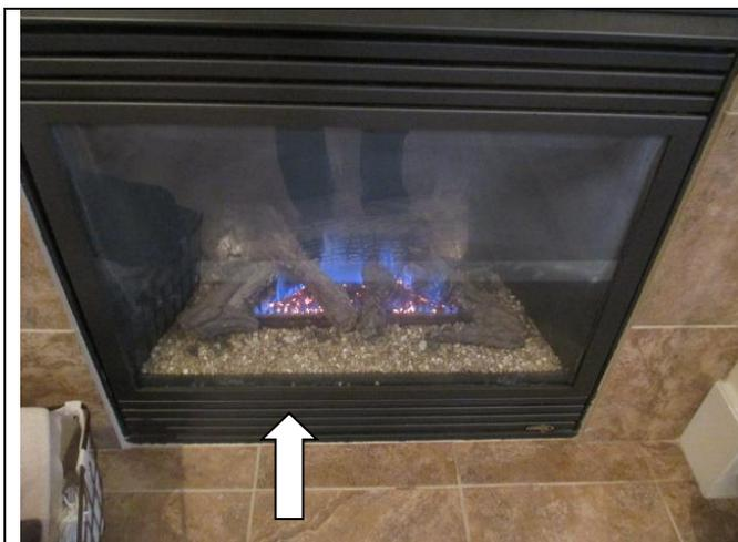
Generally the ignition components, gas shut off valve and instructions are located behind an access panel below the fireplace.
