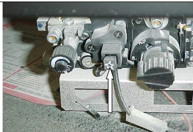
Two types of ignitor buttons are shown here. You can test the ignitor buttons prior to turning on the pilot. You should see a blue spark in the fireplace (near the pilot gas supply orifice) each time the button is pressed. If you cannot see the spark, try turning off the lights in the room.
