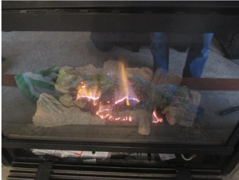
Many newer homes have a fireplace insert with gas logs installed instead of wood burning fireplaces. These generally have a wall switch to activate the full flame once the pilot light is lit. These pilot lights are considered “standing pilots” because they remain lit as long as the gas supply is turned on and do not have to be re-ignited each time the fireplace flame is used.
