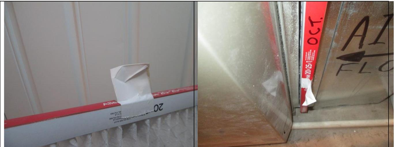
Some filters fit into the duct work without providing an edge to grasp for removal. I recommend using a piece of duct tape on the end which will provide a tab to grasp for easier removal.
