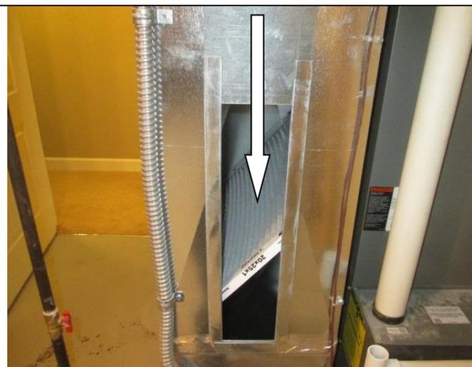
Some filters are installed diagonally and the airflow is down the return ductwork in the vertical direction.
