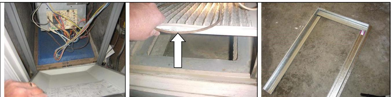
With an up-flow furnace, the filter can be located in the blower motor cabinet.
