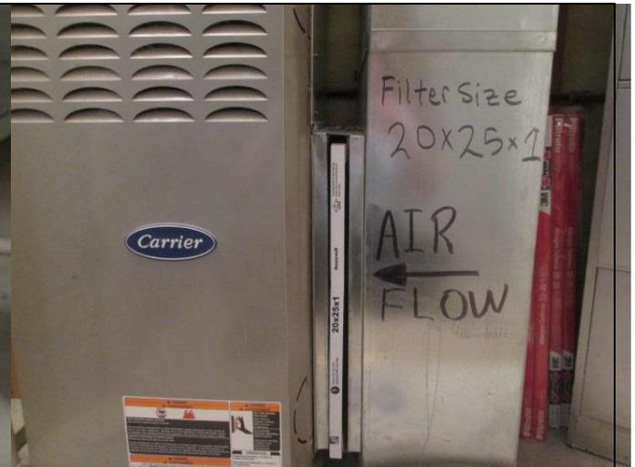
We recommend writing the air filter size and air flow direction on the side of the duct near the filter for ease of use. This filter is next the blower motor housing and the arrow should point towards the unit horizontally.
