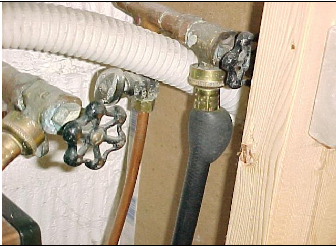
This photo shows a rubber washer hose that has expanded and is about to fail.
